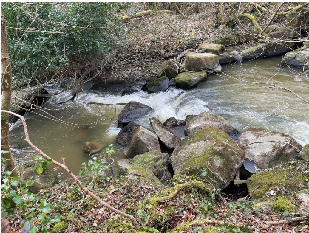
Figure 7: View of boulder weir, February 2026
