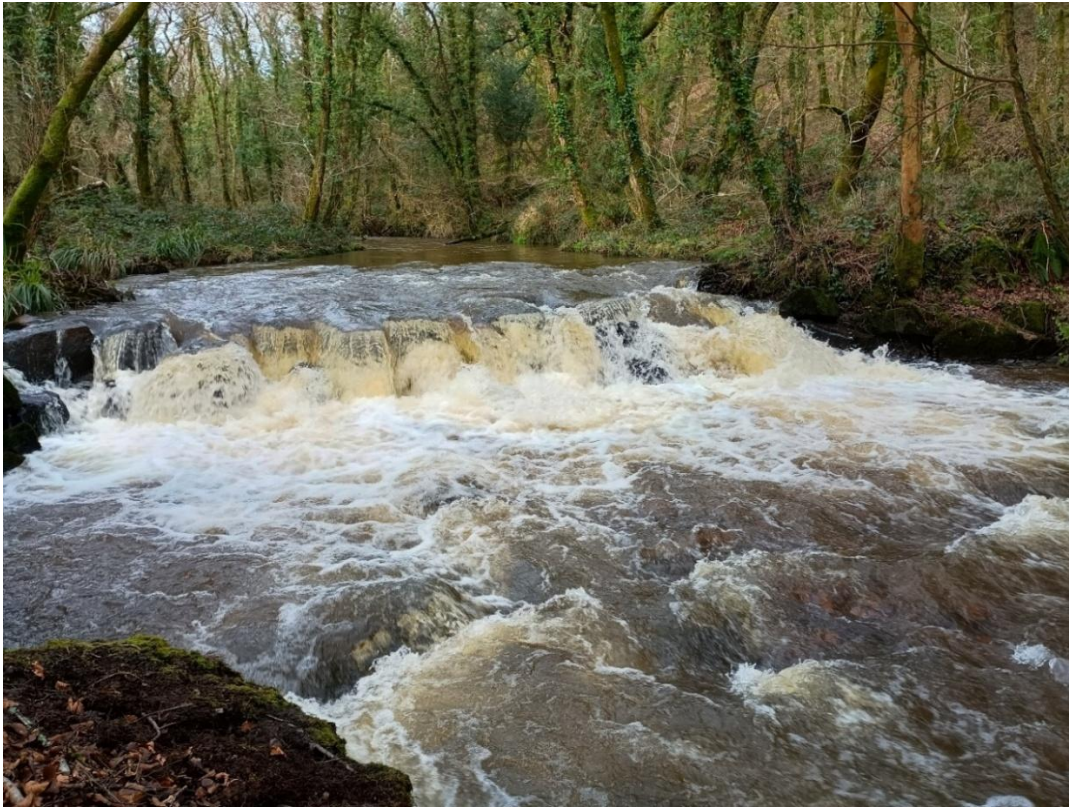
Figure 110: Treviscoe Weir from downstream, February 2026
