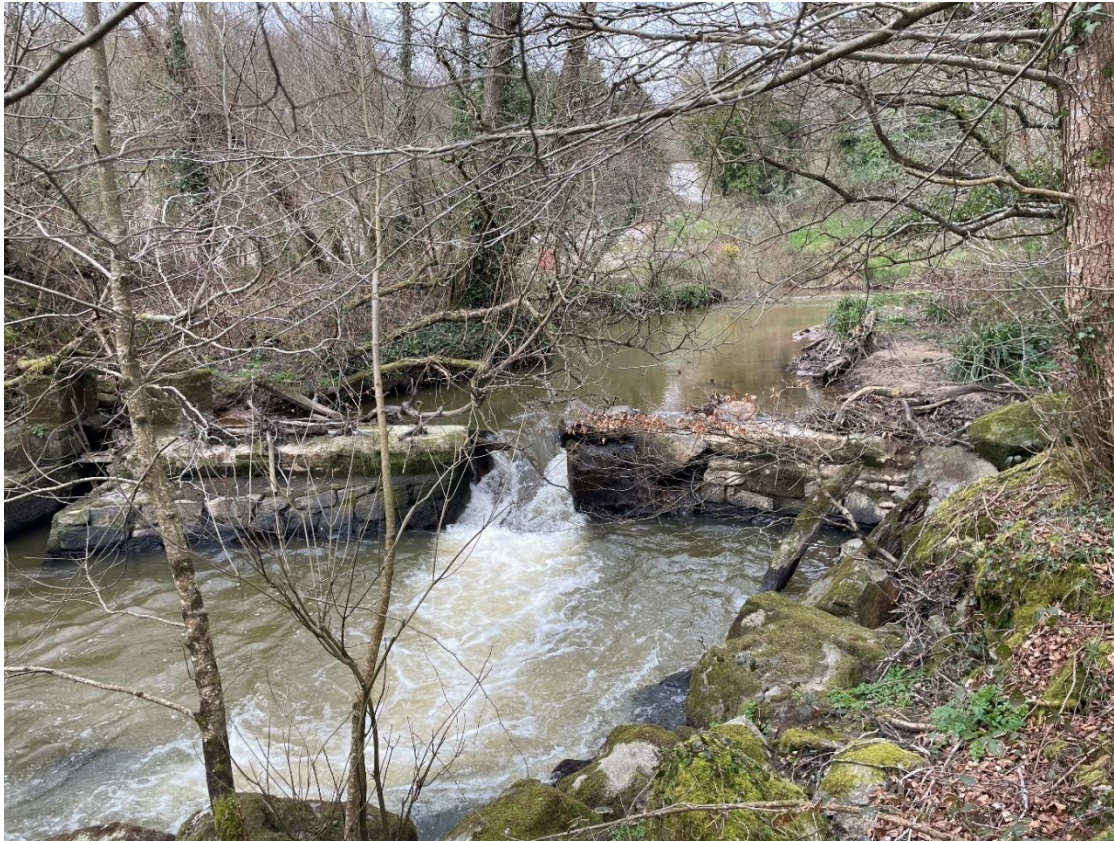
Figure 8: View upstream to structure, February 2026
