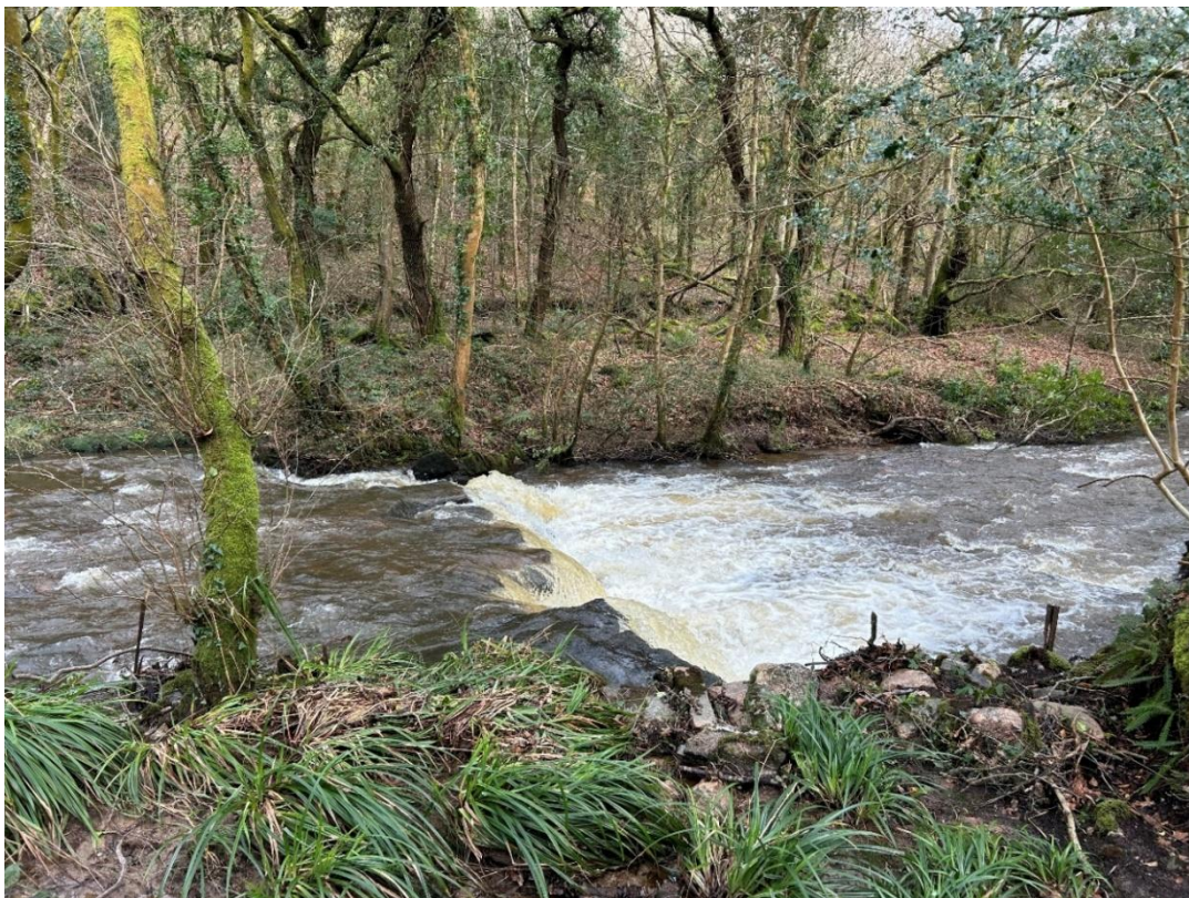
Figure 101: View to Treviscoe weir from right hand bank, February 2026
