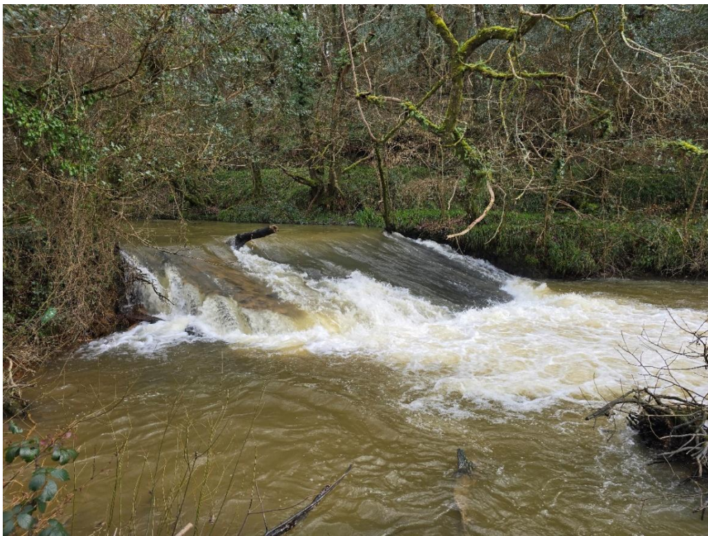
Figure 3: Trenowth Weir from right bank, February 2026
