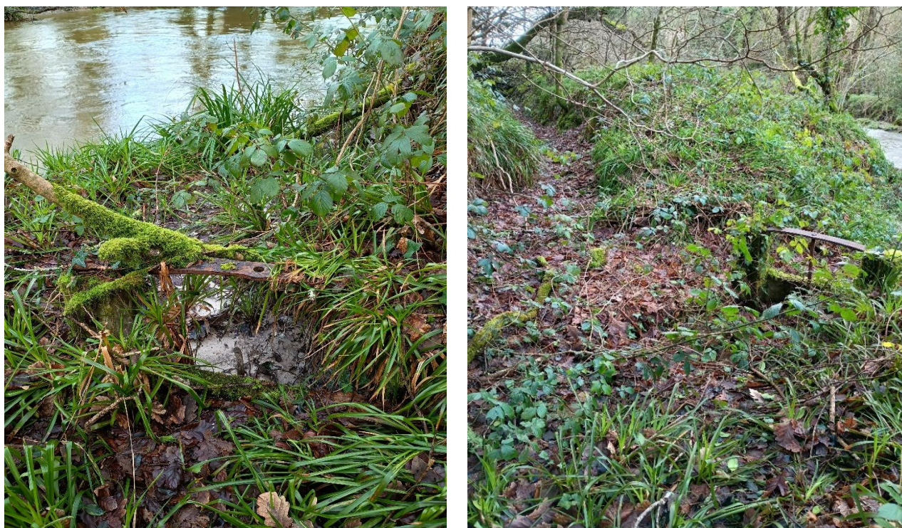
Figure 4: Trenowth Weir leat sluice gate inlet (left) and outlet (right), February 2026
