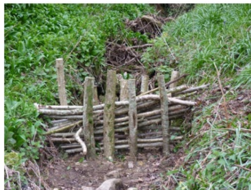
Leaky barrier using hazel bundles
