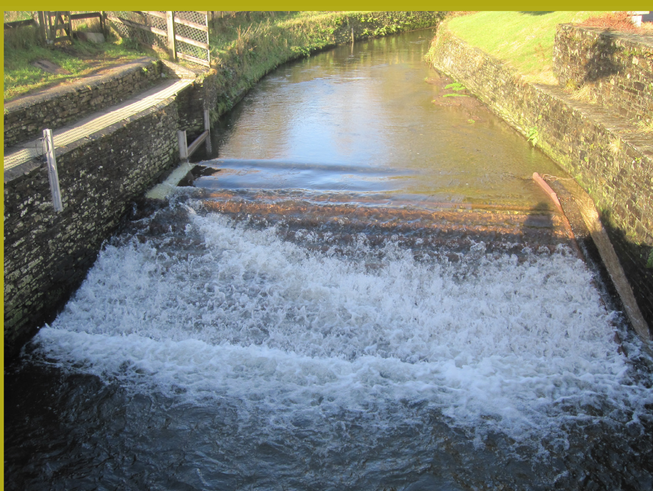
After - Camelford weir: Baffled weir face and flow control structure at redundant fish pass entrance (left) with bristled eel pass on the right hand side.
