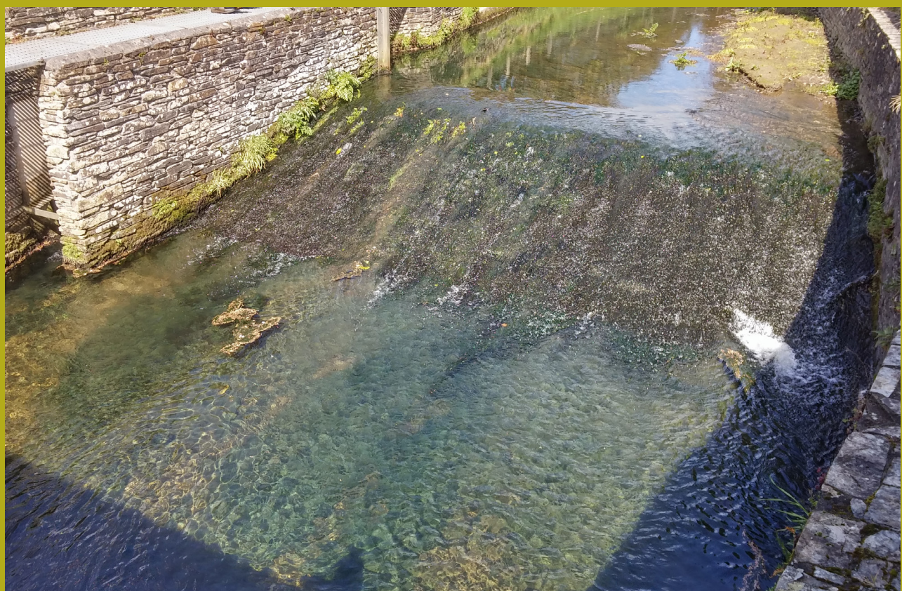
Before - Camelford weir: A damaged weir face (bottom right) and a poorly functioning technical fish pass on the left.
