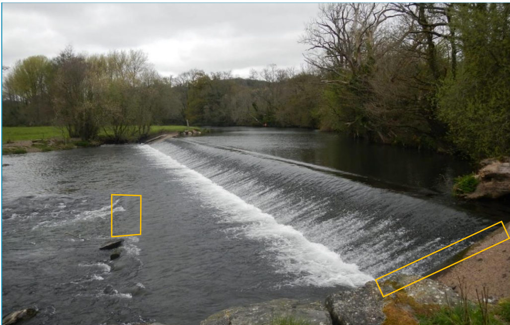
Photo 5: Bolham weir from the true left-hand bank. Yellow box indicates the proposed location for a smolt chute and downstream notch.
