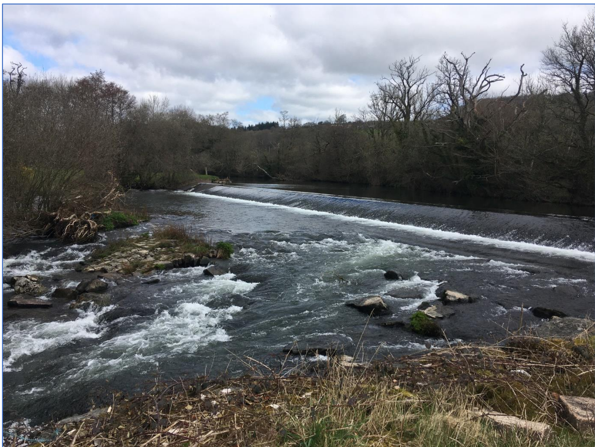
Figure 3. The downstream end of the barrier in low flows
