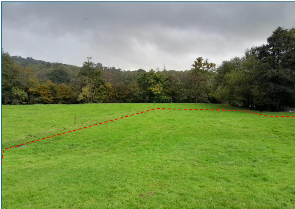
Photo 21: Looking towards the RHB and the area for the construction of the fish pass. (Temporary site compound marked by red dashed line).
