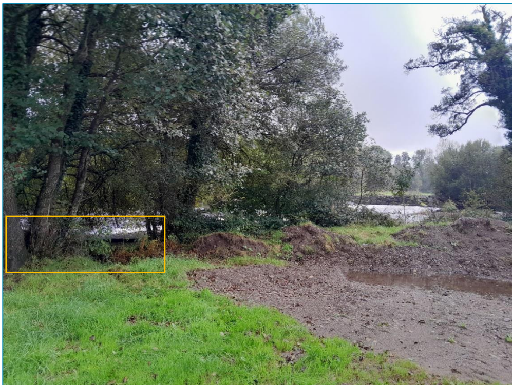
Photo 2: Yellow box indicates the location of the downstream end of the proposed fishpass and weir stilling basin several trees here will need to be thinned but canopy should remain for shading and cover from predation.
