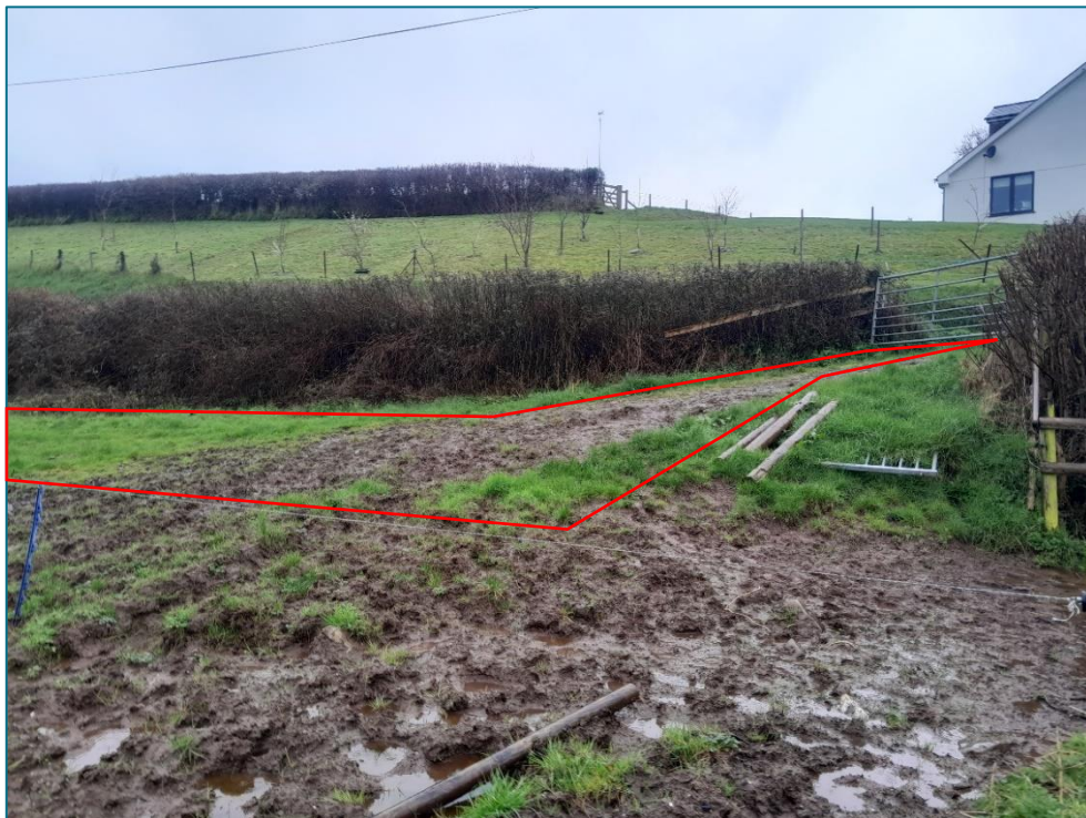
Photo 7: The start of the turnaround area and entrance to the permanent access track. Area for turnaround marked by a Red box.
