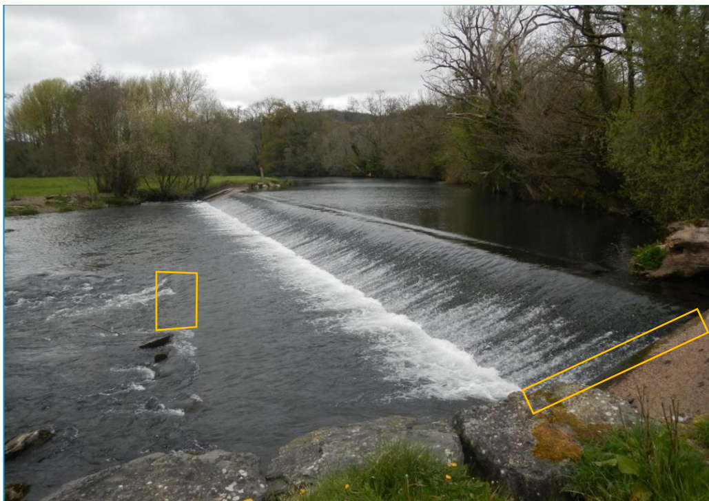
Photo 5: Bolham weir from the true left-hand bank. Yellow box indicates the proposed location for a smolt chute and downstream notch.
