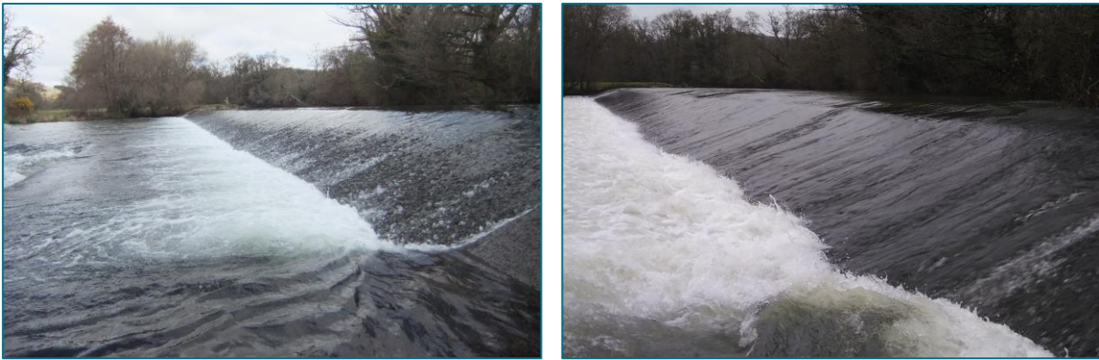
Plate 1: Bolham weir under different flow conditions. Left: Q45 flows revealing water depth on weir face still very shallow under prime migratory flows. Right: Q10 flows revealing strong laminar flows presenting challenging swimming conditions for all but larger more capable salmonid specimens.
