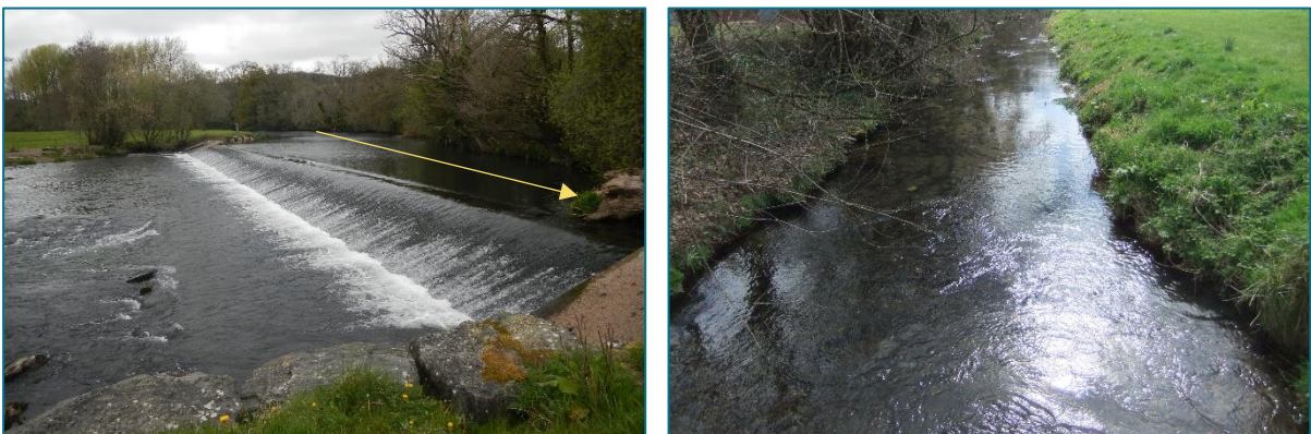
Plate 2: The weir actively directs downstream migrating fish to the leat offtake (left) which may increase risk to downstream migrating fish. For example, easy access for wading avian predators and lack of cover (right).
