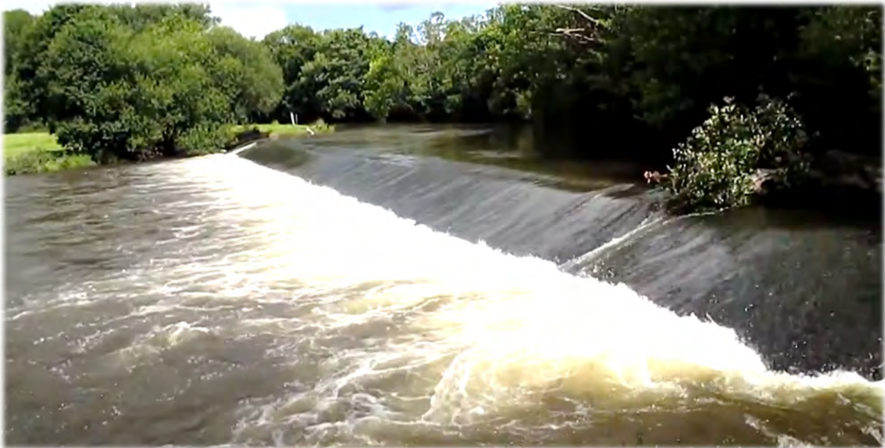
Figure 3: Bolham Weir Structure (looking north). Source: David Jury, 2020, YouTube.com
