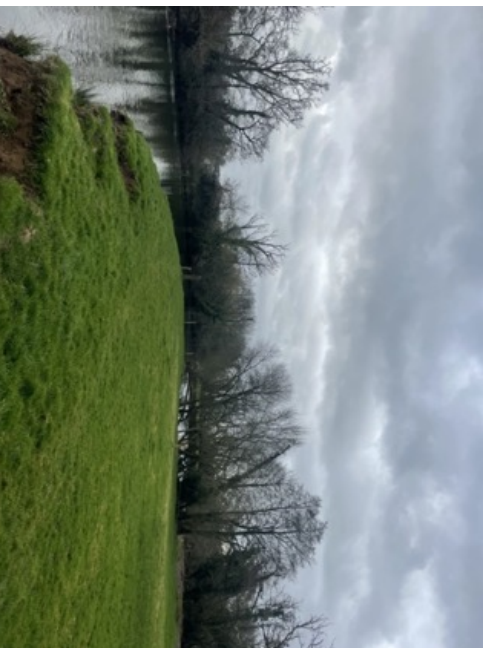
Downstream view of weir and scattered trees at true right bank, bordered by grassland
