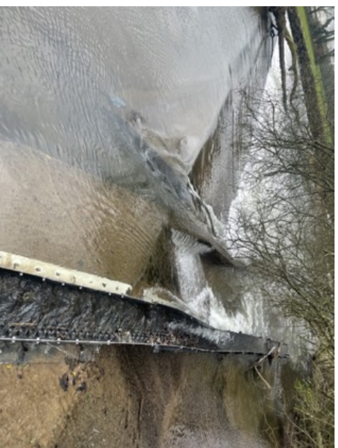
Existing eel pass and redundant fish pass at true right bank
