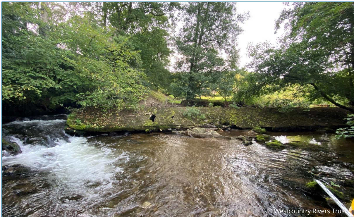
Plate 1: Looking north (upstream). View of the weir and breach on the RHB.
