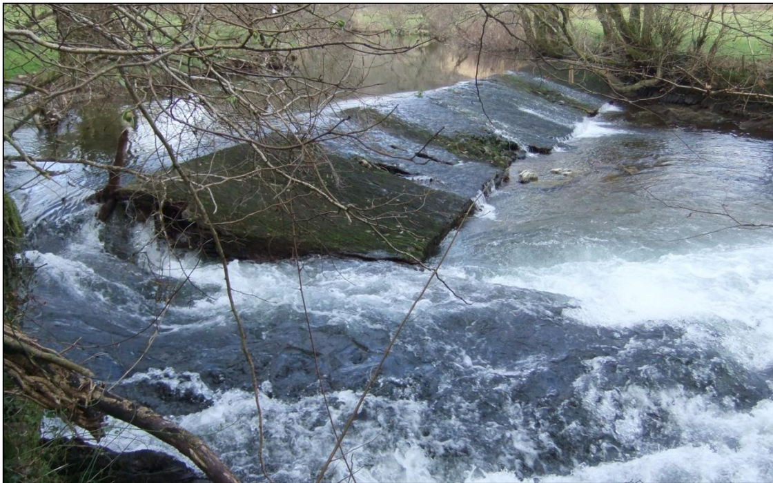
FIGURE 9: PHOTOGRAPH 2020/2021 BY WESTCOUNTRY RIVERS TRUST PERSONNEL, FROM THE WEST BANK – SHOWING DAMAGE TO THE WEST END OF THE WEIR.
