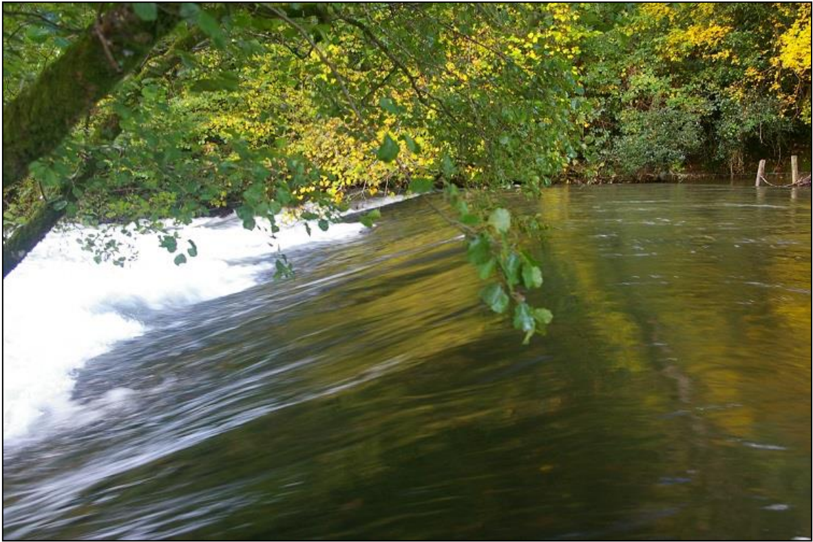
FIGURE 8: VIEW ACROSS THE WEIR, SHOWING THE PROFILE OF ITS CRUMP FORM; FROM THE EAST.
