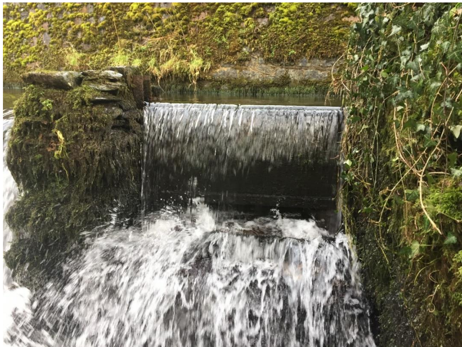
Figure 2.7: Image of the notch (with boards inserted) at the downstream end of the weir, close to the sluice at the head of the leat
