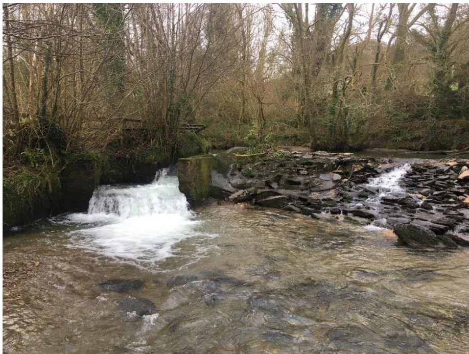
Figure 2.3: image of the fish pass at the upstream end of the weir, looking from downstream
