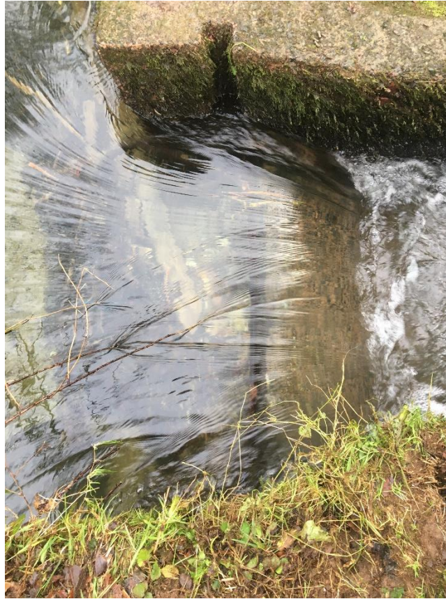
Figure 2.4: Image of the upstream end of the fish pass, where flow enters the pass. Boards are typically placed in here, to reduce flow into the pass
