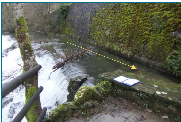
Plate 2: The weir actively directs downstream migrating fish to the leat (left) where mill infrastructure has high potential of causing damage (example: right)
