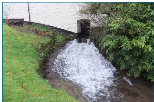
Plate 2: The weir actively directs downstream migrating fish to the leat (left) where mill infrastructure has high potential of causing damage (example: right)
