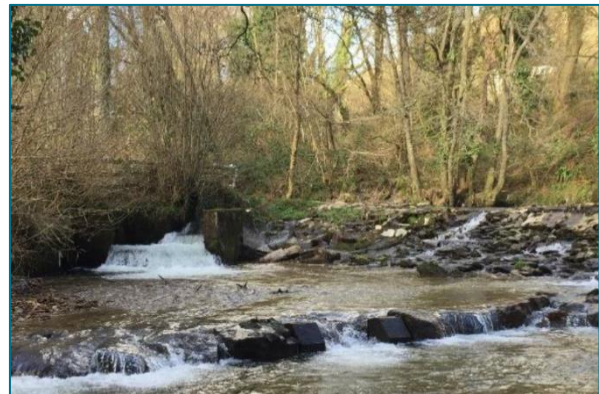
Plate 1: The combination of the existing fish pass (left) and pre-barrage installed in 2012 as a temporary measure (right) is still restricting access for protected native migratory fish species.
