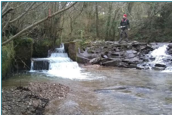
Plate 1: The combination of the existing fish pass (left) and pre-barrage installed in 2012 as a temporary measure (right) is still restricting access for protected native migratory fish species.
