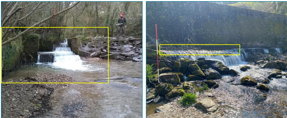
Plate 3: Left: Existing channel to house new technical fish pass, area to be excavated to produce a larger pool, section of wall to be removed to accommodate new fish pass, and area of extended weir toe with stone. Right: Area of crest to be raised to reduce competing attraction flow.
