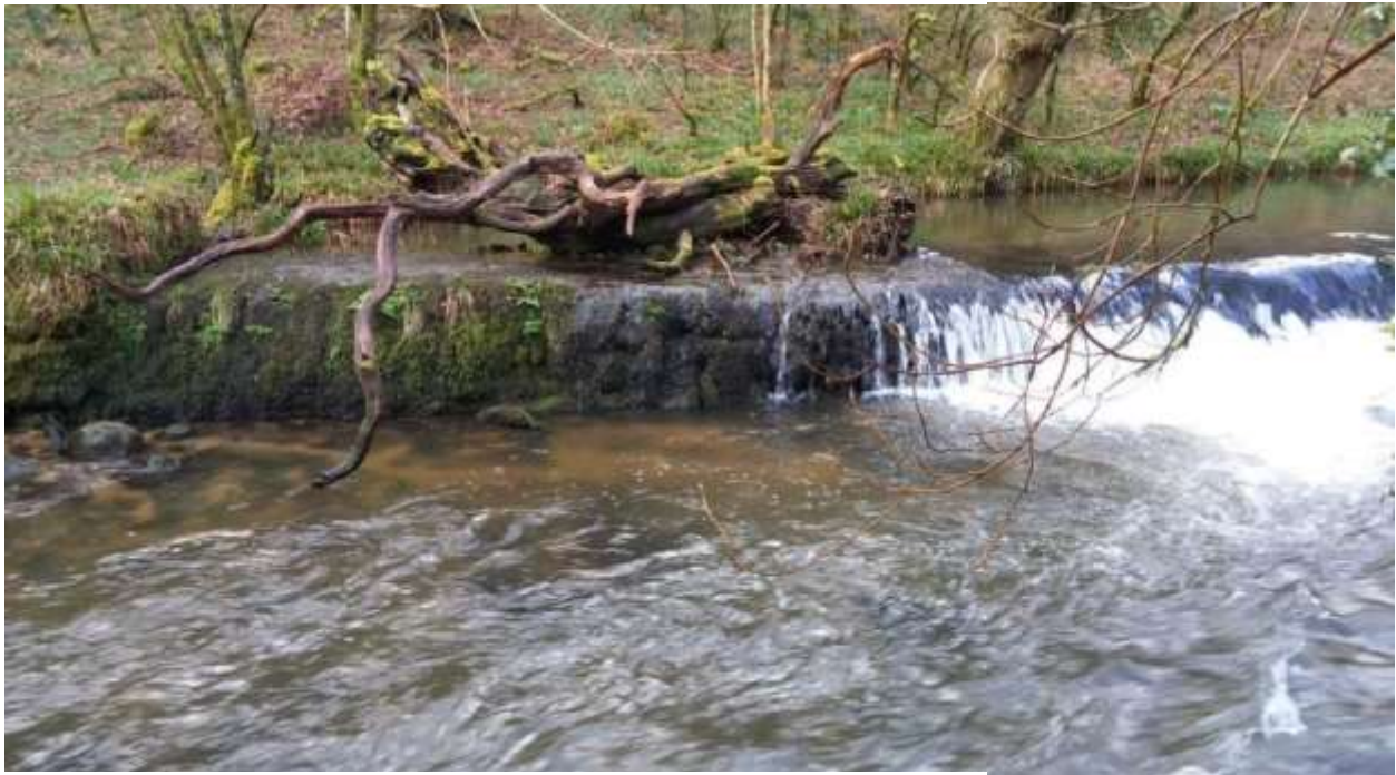
Photo 3: View of left-hand side of stone structure face
